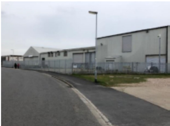
Former abattoir site, Heath Road, Skegness
